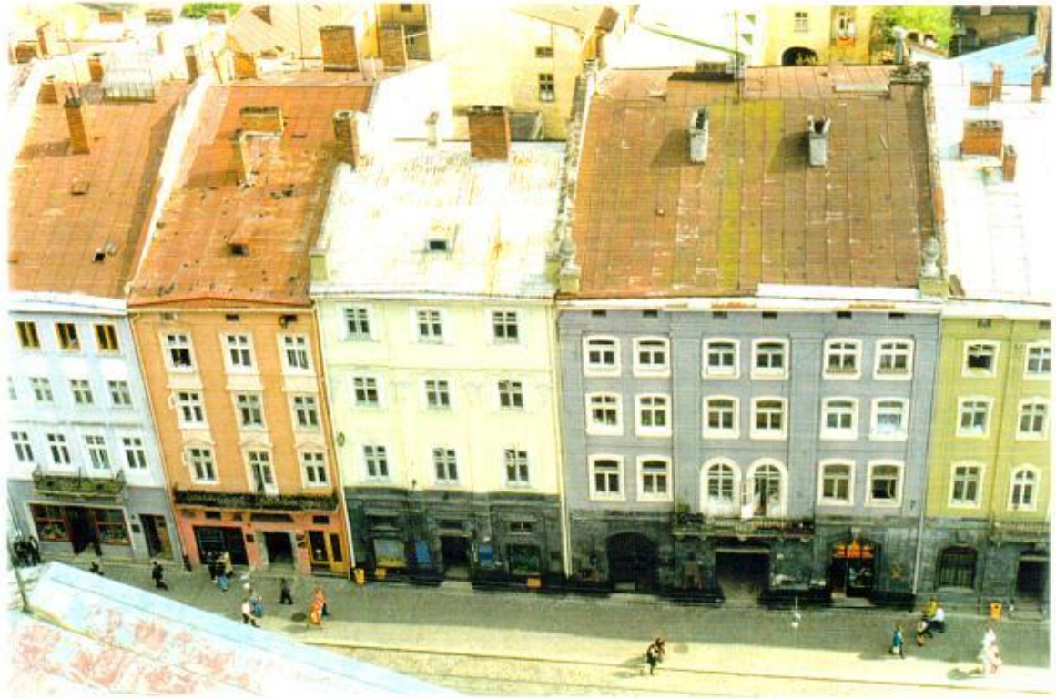
19. RYNOK SQUARE: BUILDINGS ON THE SOUTH SIDE, 16th-20th c
